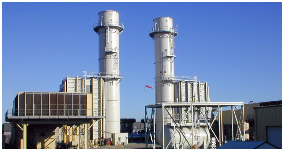
Two GE Frame 7 turbines with Johnson Matthey SCR/CO Catalyst systems.
